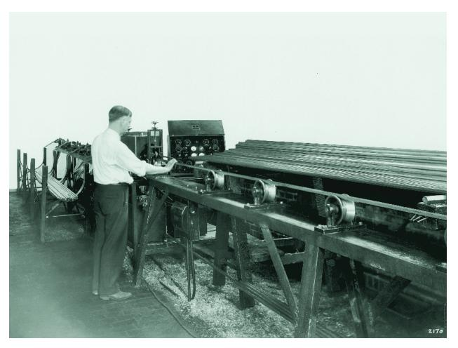
In 1934, Union Drawn Steel became the first company to install Magnetic Analysis Corp's electromagnetic tester. The concept of an operating lease for NDT equipment was launched and remains a successful part of MAC's<sup>®</sup> marketing program today.
