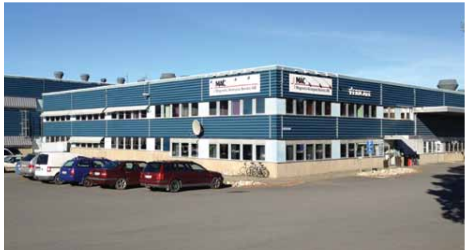
Magnetic Analysis Nordic's plant in Östersund, Sweden is one of MAC's three manufacturing plants.
